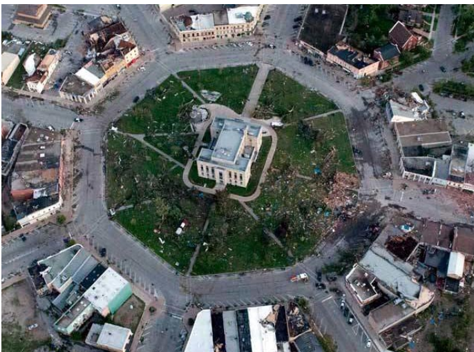
Destruction Caused to West Street, The Square and Court House, Goderich, Ontario, August 21, 2011.
