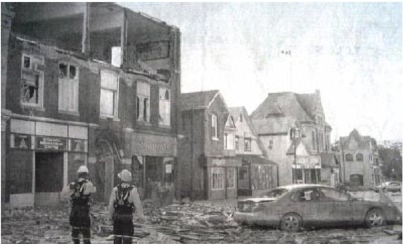
The Top of West Street Showing the Destroyed Façade of the Masonic Building and Rubble Strewn Across the Road. A Scene Reminiscent of a War Zone.
