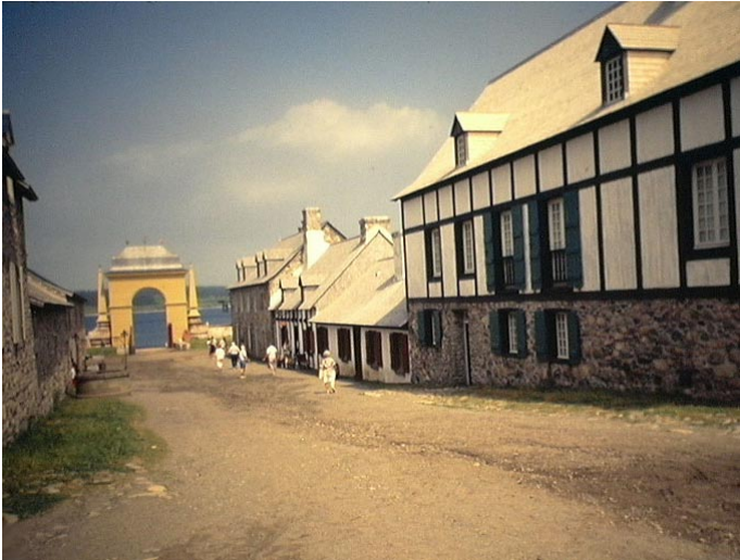
Rue Principale (Main Street) in the Reconstructed Fortress Louisbourg, Nova Scotia, August, 1989.
