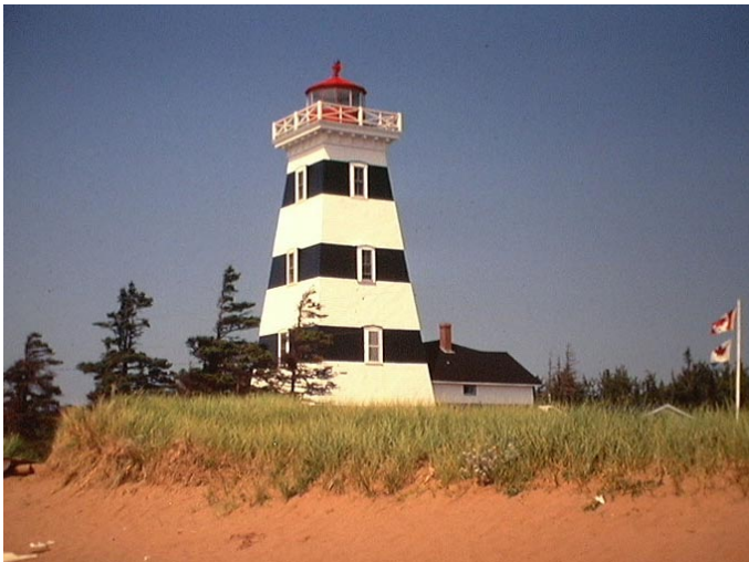
West Point Lighthouse, now Part of an Inn, Western Region of Prince Edward Island, August, 1989.
