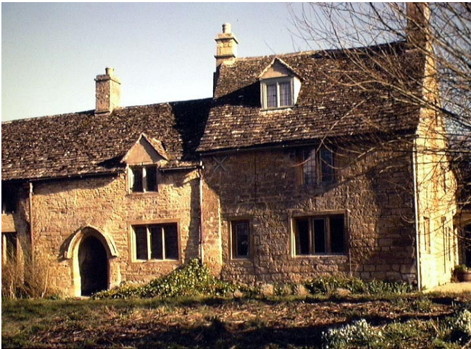
Typical Cottages Made from Cotswold Stone at Little Barrington, England, March, 1994.
