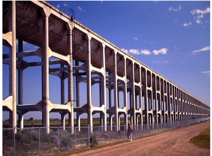
Reinforced Concrete Pillars Supporting the Brooks Aqueduct, Brooks, Alberta, July, 1994.
