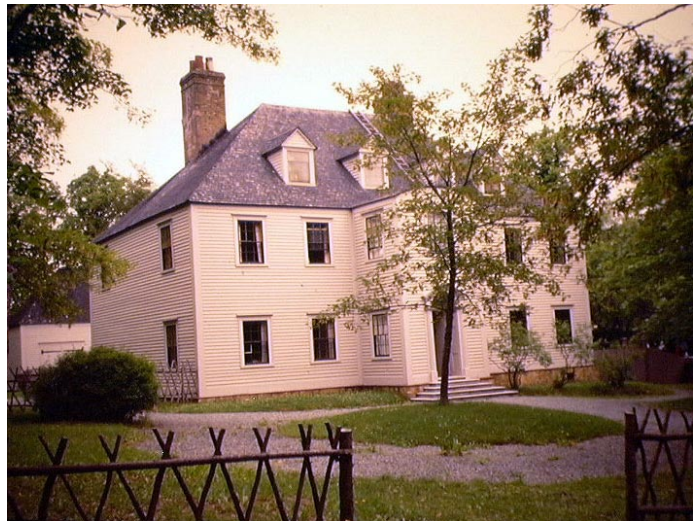
Commissariat's House, one of the Preserved Historic Buildings in St. John's, N.L., July, 1995.
