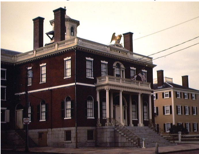
The Salem Maritime National Historic Site Custom House, Salem, Massachusetts, July, 1997.
