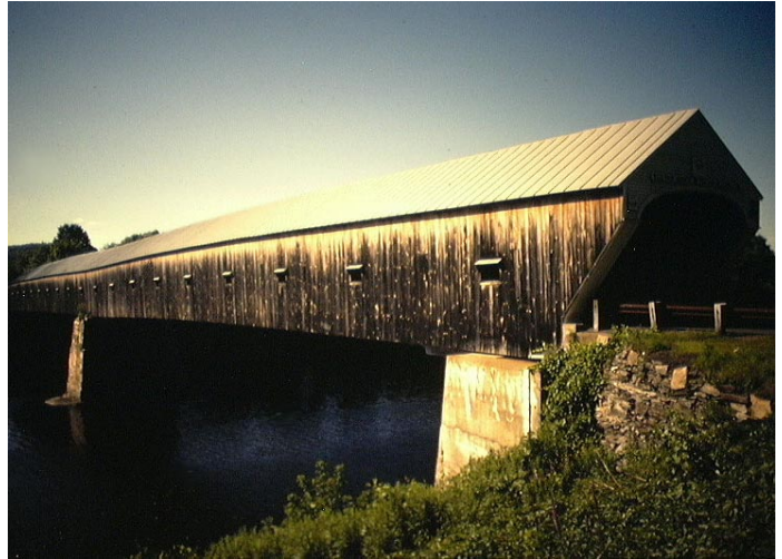
The Windsor-Cornish Covered Bridge. Longest in the U.S.A., New Hampshire, August, 1997.
