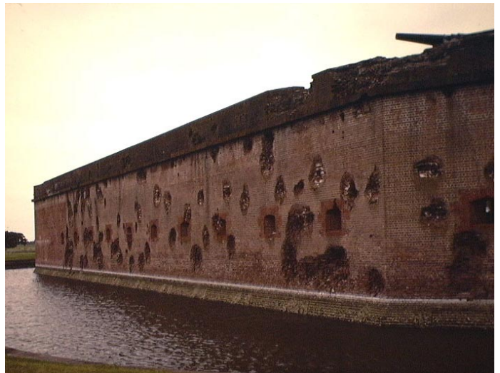
Battle Scarred Brick Walls of Fort Pulaski, Georgia, April, 1998.
