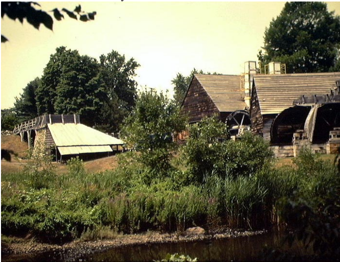
General View of the Saugus Iron Works National Historic Site, Saugus, Massachusetts, July, 1997.
