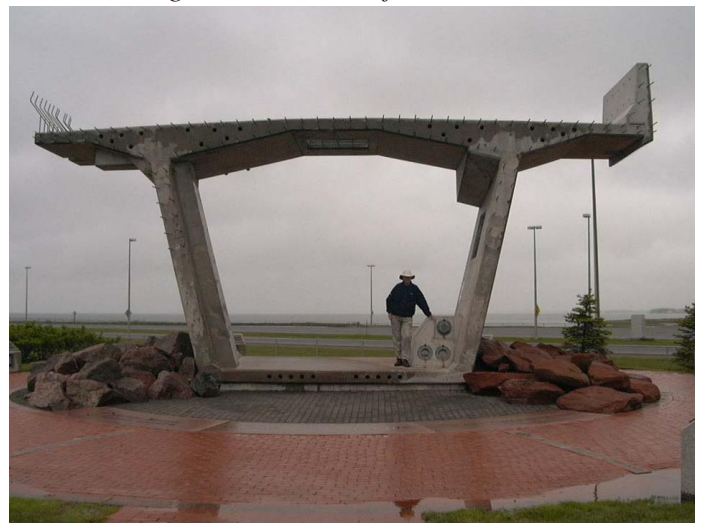
Barry Poses with the Static Exhibit of a Cross-Section of the Confederation Bridge, NB/P.E.I., June, 2003.
