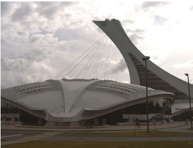
Exterior of the Olympic Park with the Stadium Tower and Vélodrome, Montréal, Québec, July, 2004.
