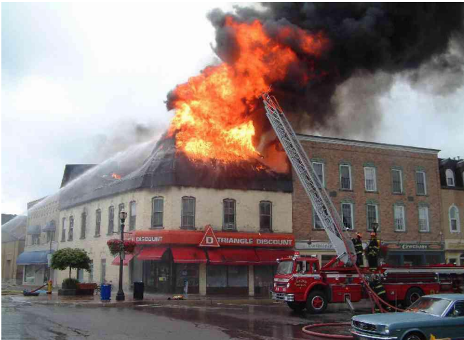
Fire Erupts at the Triangle Discount Store on North Street and The Square, Goderich, ON, July, 2004.
