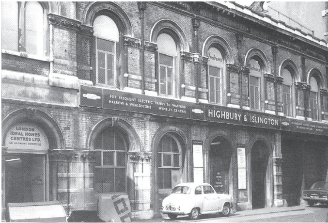
Highbury & Islington Station Forecourt, 1950
