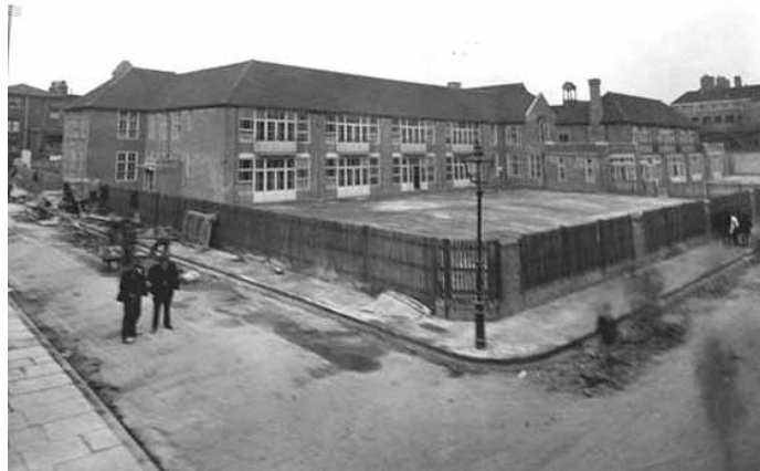
Barnsbury Secondary School for Boys (Lower School), Geary Street at Georges Road, Islington, c1931
