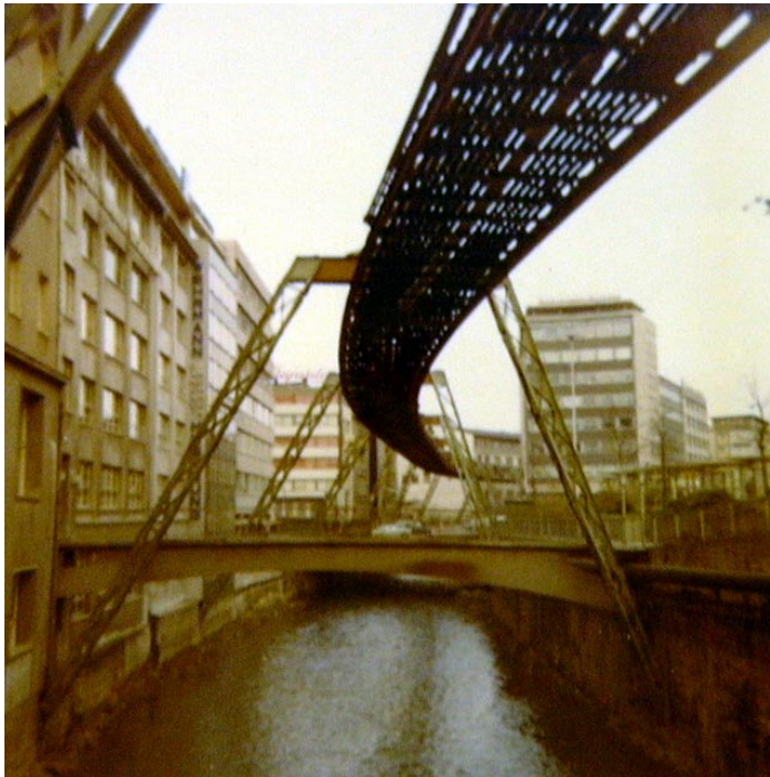
Length of Track of the Suspended Monorail Railway (Schwebebahn), Wuppertal, Westphalia, Germany, 1966.
