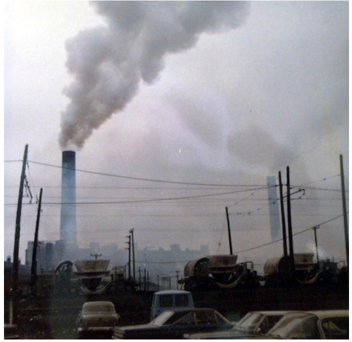
The Two Chimneys of the INCO Nickel Smelter. In the Foreground are the Hopper Cars Carrying Hot Slag that is Discharged on the Tailing Piles, Sudbury, Ontario, Canada, 1967.
