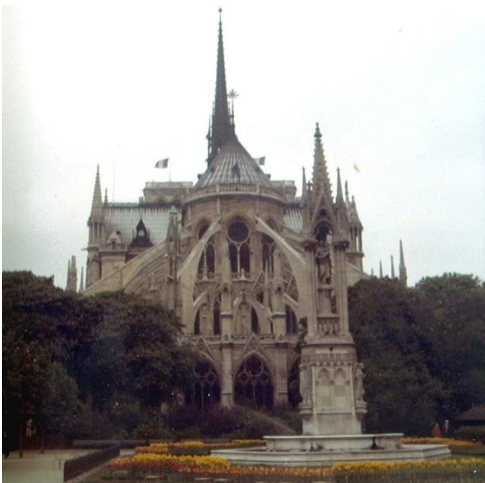
Rear View of Notre Dame Cathedral Showing the Impressive Flying Buttresses, Île-de-la-Cité, the Historical Heart of Paris, France, April, 1972.
