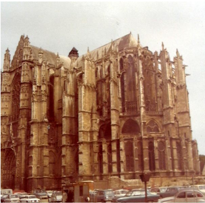
Southeast View of the Cathedrale de Saint Pierre Showing the Massive Gothic Flying Buttresses, Beauvais, near Paris, France, April, 1972.
