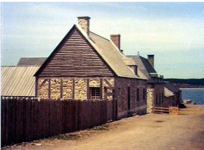
Reconstructed Houses, Fortress of Louisbourg National Historic Site, Nova Scotia, June, 1975.
