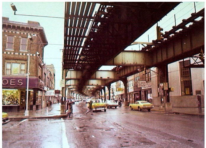
Elevated Section of the New York Subway System, Jamaica Road, Queens, New York City, March, 1975.
