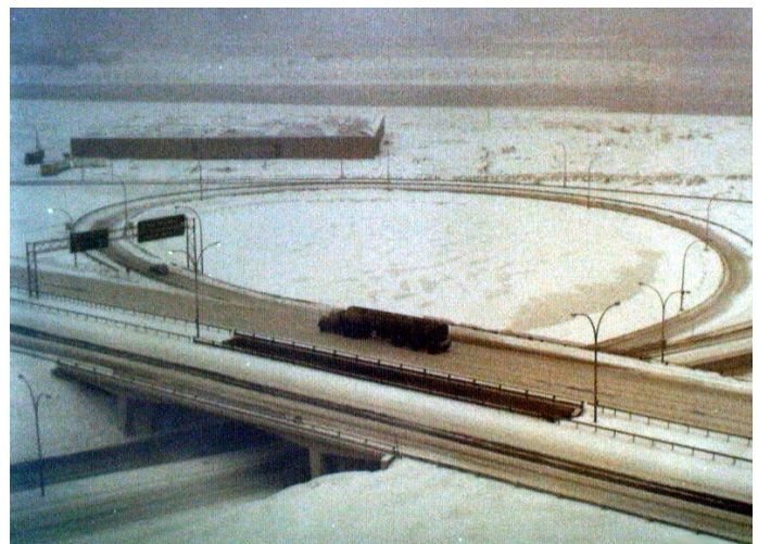
Overlooking the Taschereau Boulevard Interchange During a Blizzard, Longueuil, Québec, Jan., 1975.
