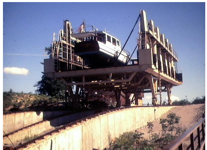
Marine Railway Transporting Pleasure Craft on the Severn River, Big Chute, Ontario, August, 1979.
