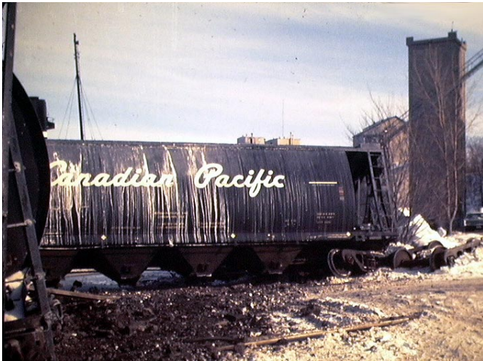
Derailed CPR Tanker Cars and Spilled Salt Cargo, Goderich, Ontario, January, 1978.
