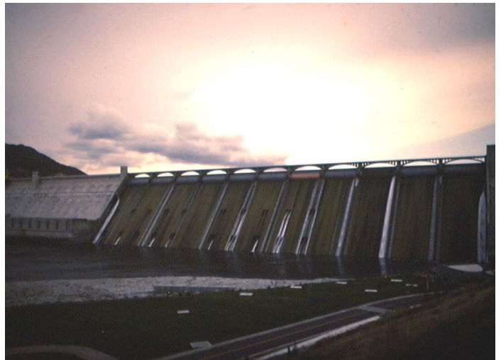
Grand Coulee Dam, 1930s Depression Work Project, Washington, U.S.A., May, 1981.
