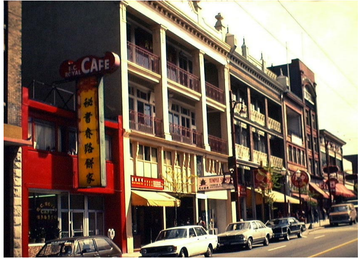
Typical Buildings in the Ethnic Chinatown District of Vancouver, BC, May, 1981.
