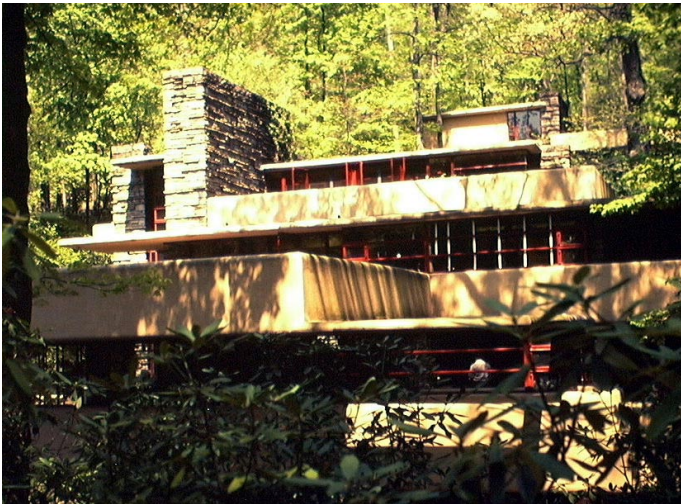
Exterior of "Fallingwater" Designed by Frank Lloyd Wright, Bull Run, Pennsylvania, May, 1981.
