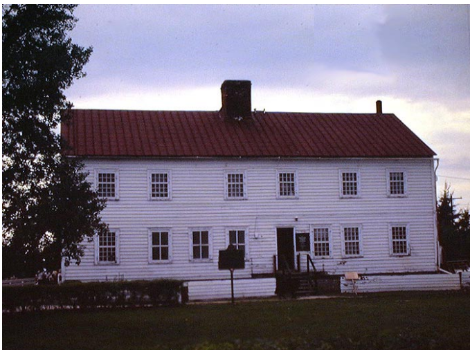
Hudson's Bay Company Trading Post (Factory), Moose Factory Island, Northern Ontario, July, 1980.
