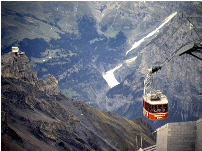
The Schilthorn Cable Car Seen from the Summit of Mount Schilthorn, Switzerland, September, 1982.
