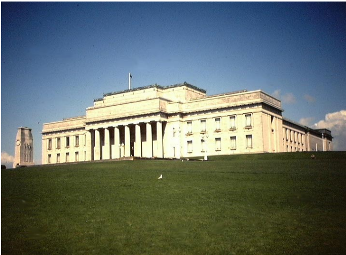
Exterior of the New Zealand War Museum with the Cenotaph, Auckland, New Zealand, March, 1984.
