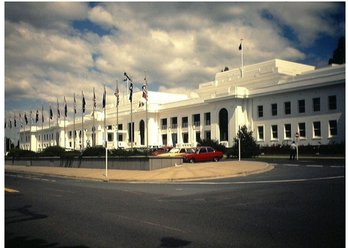
Detail of the Federal Provisional Parliament House in Canberra, Australia, February, 1984.
