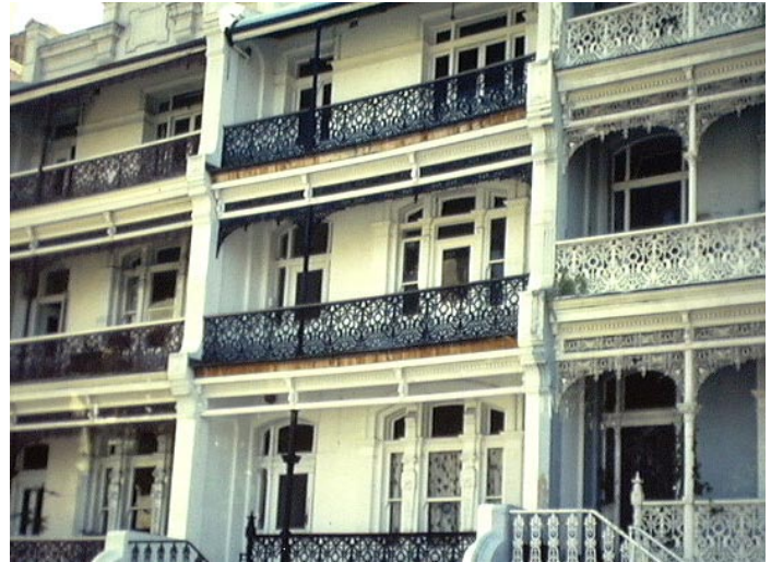
Paddington Terrace Houses with Ornate Wrought Iron Balustrades, Sydney, Australia, March, 1984.
