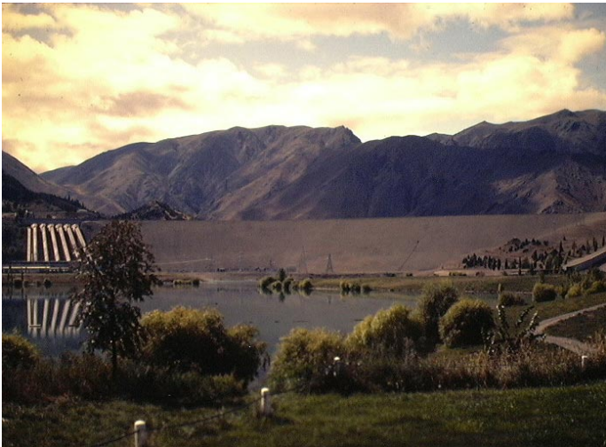
View of the Benmore Dam near Twizel, South Island, New Zealand, March, 1984.
