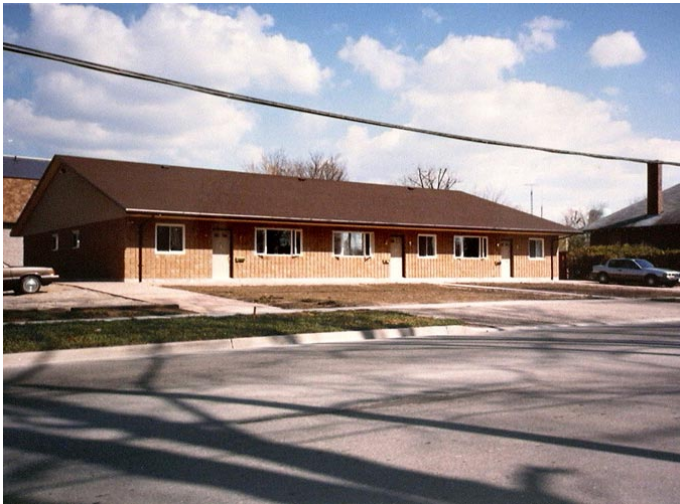
Exterior of the Cambria Road Apartment Building, Goderich, Ontario, March, 1987.
