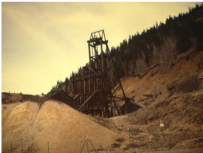
Abandoned Gold Mine Headframe with Slag Heap Tailings near Cripple Creek, Colorado, May, 1987.
