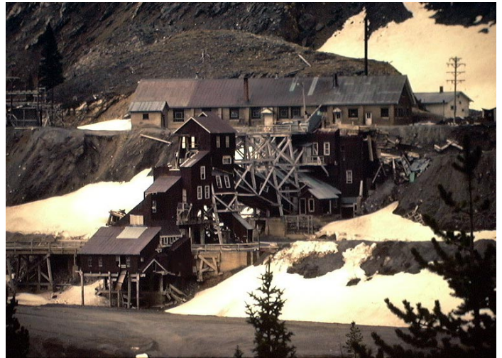
Working Gold Mine Headframe and Mill Buildings, near Monarch Pass, Colorado, May, 1987.
