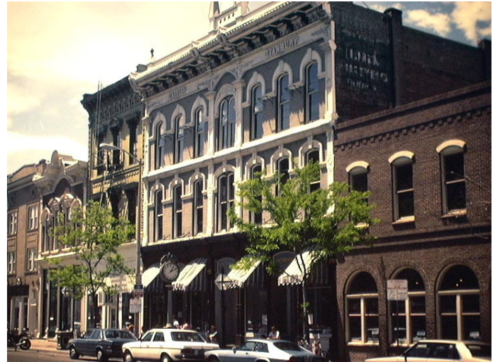
Larimer Square, Historic Part of 16th Street Mall, Denver, Colorado, May, 1987.
